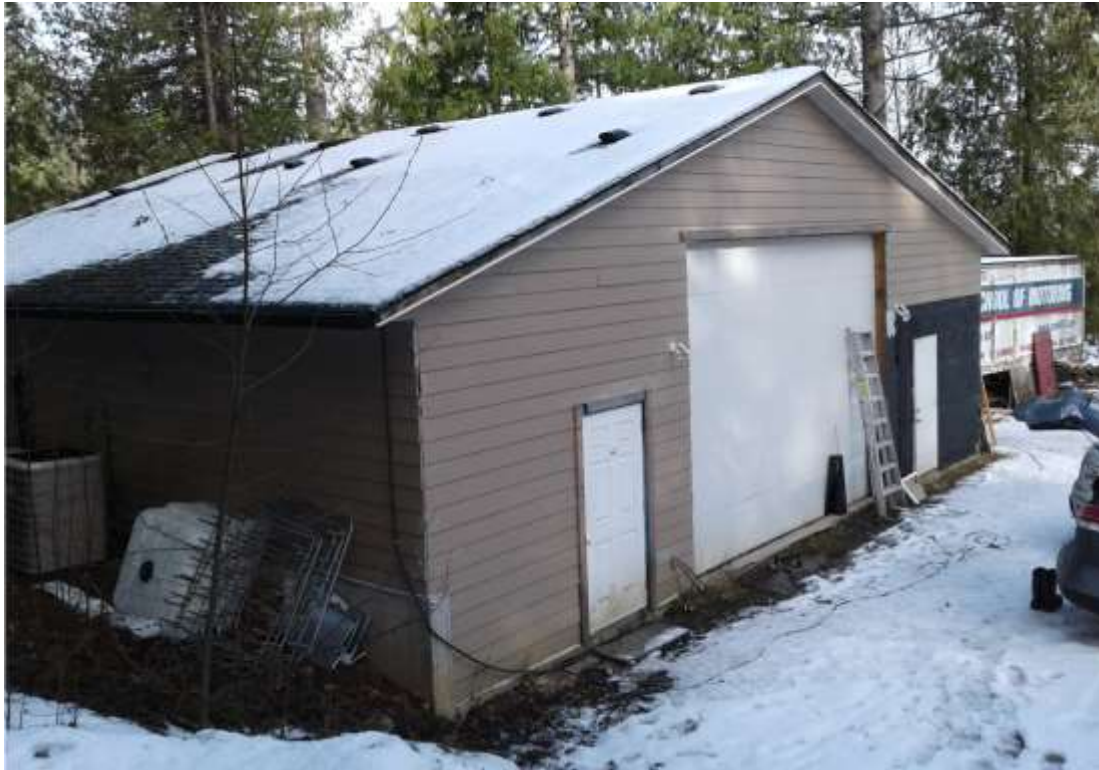
Figure 3: Front of accessory building facing into the subject property
