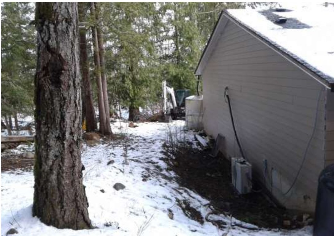
Figure 4: Rear of Accessory Building facing into the neighbouring property
